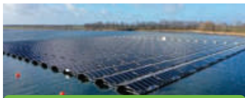
Weperpolder, NL, 2,1 MWp 2018
